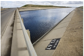
13. California Aqueduct. Westland Irrigation District. Central Valley, California. March 2009. Archival pigment print. 20 x 30 inches
